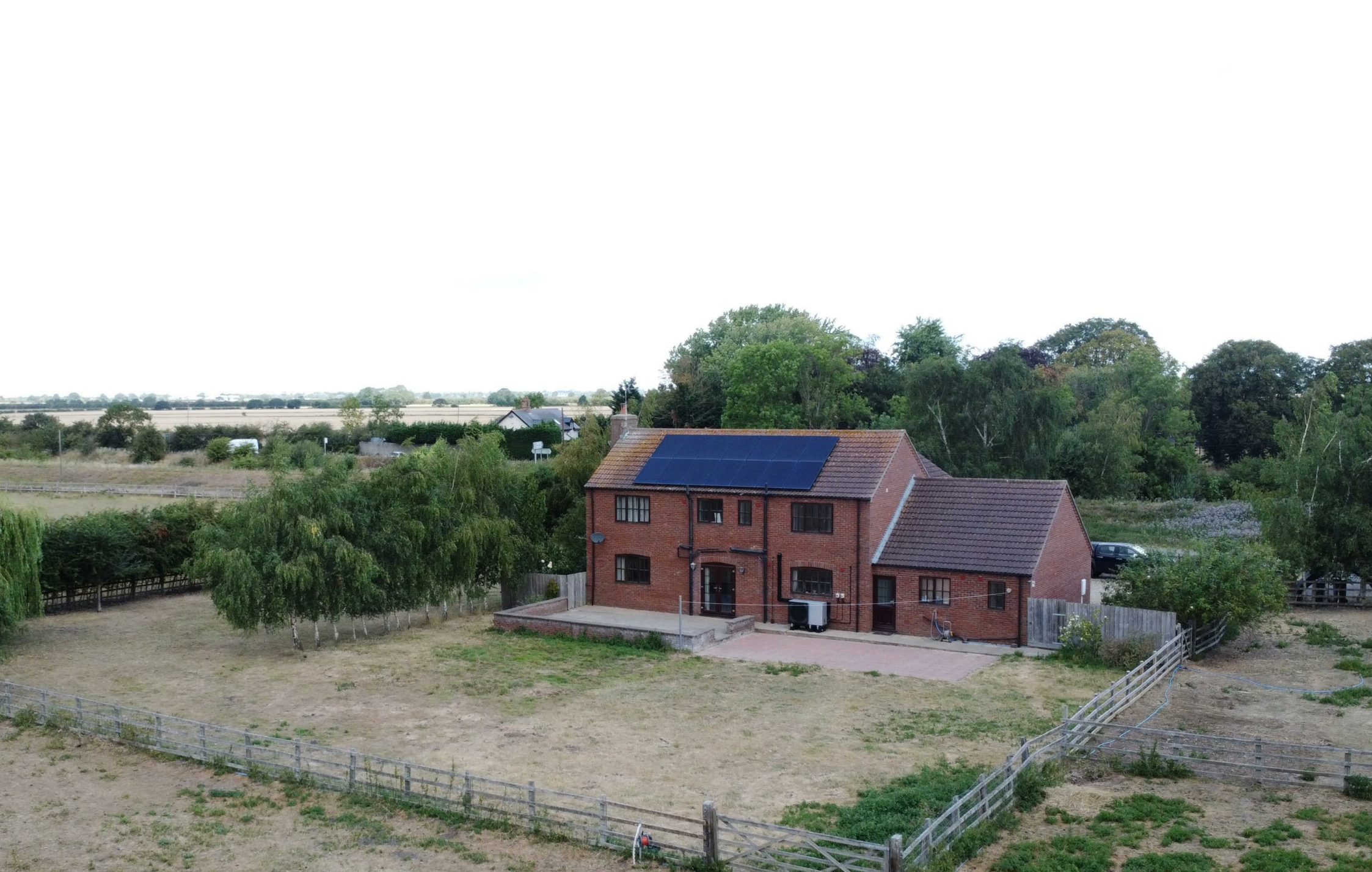
River Bank House Saxilby
